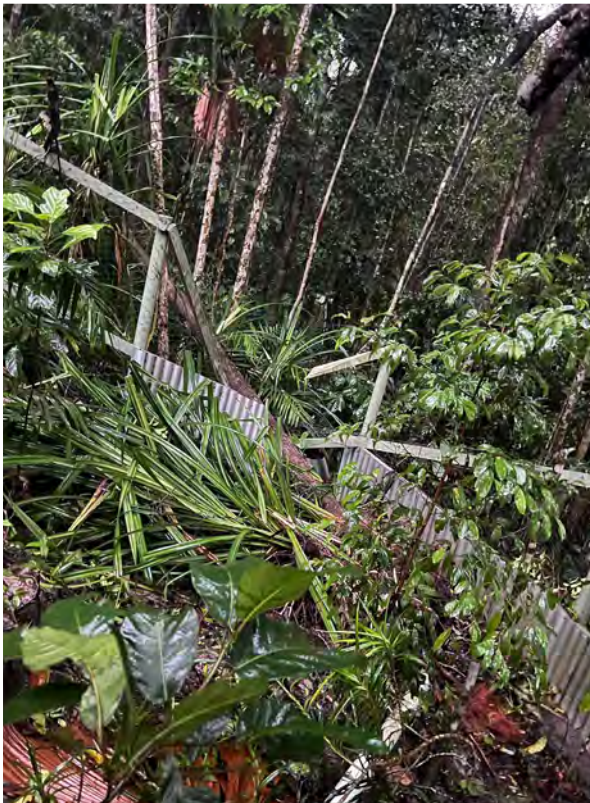
LANDSCAPE DAMAGE FROM WIND AND RAIN
