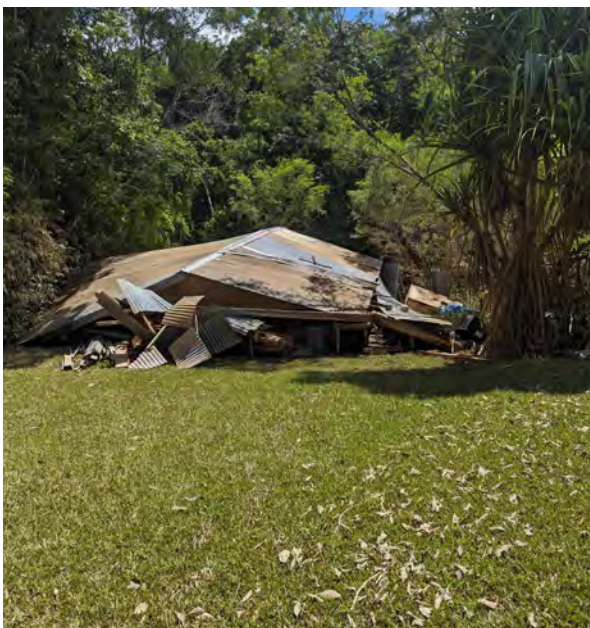
BUILDING COLLAPSE AT RUSSET PARK DUE TO FLOODING
